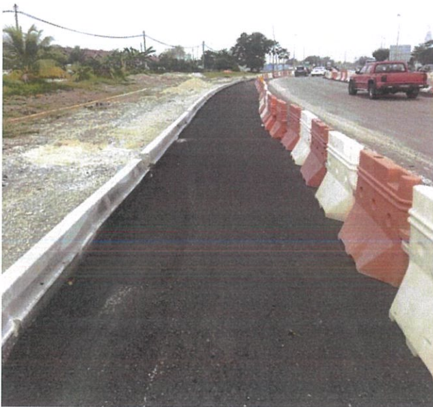
PHOTO 7: Pavement works (Binder course) in progress at CH B
