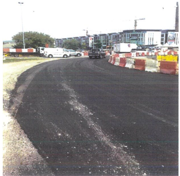
PHOTO 14: Resurface roundabout area in progress
