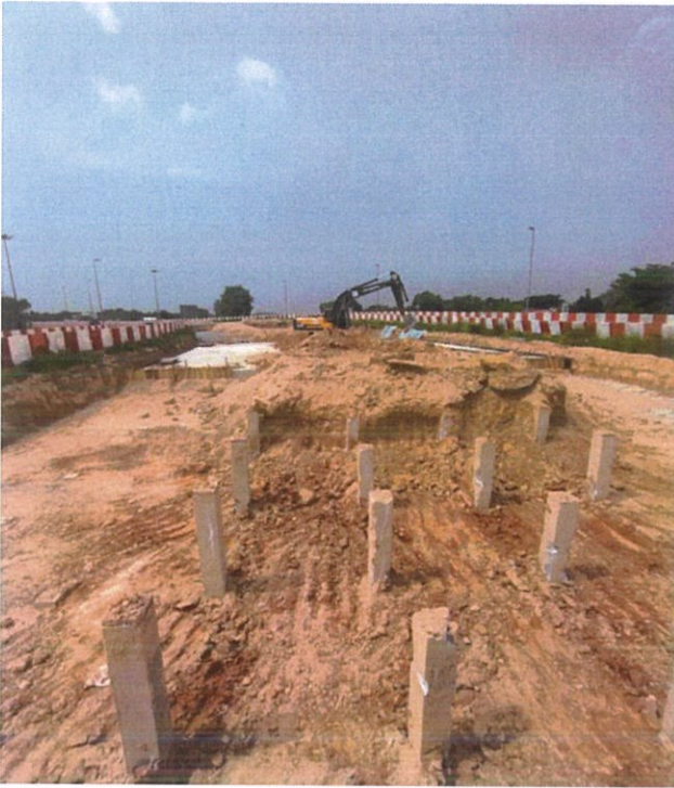
PHOTO 1: Pile Embankment - Excavation & backfilling works in progress at zone 3 SKVE
