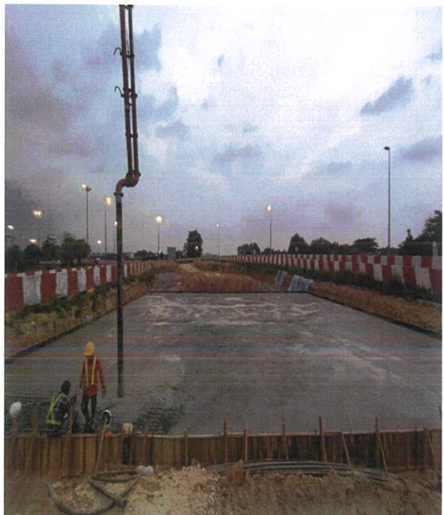
PHOTO 4: Pile Embankment - Concreting pile raft slab in progress at Zone 3 SKVE
