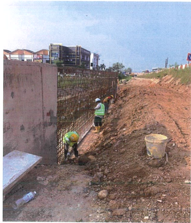
PHOTO 10: RC Wall in progress at CH E (ELITE)
