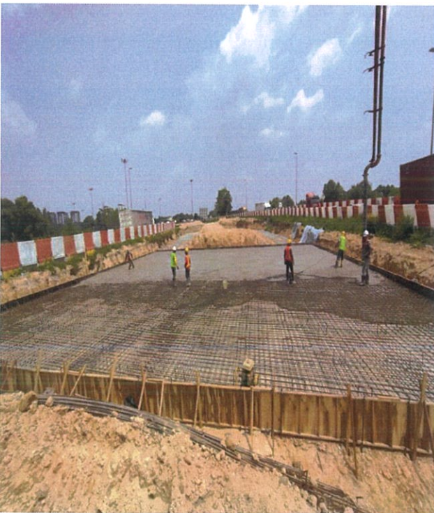
PHOTO 3: Pile Embankment - Concreting pile raft slab in progress at Zone 3 SKVE
