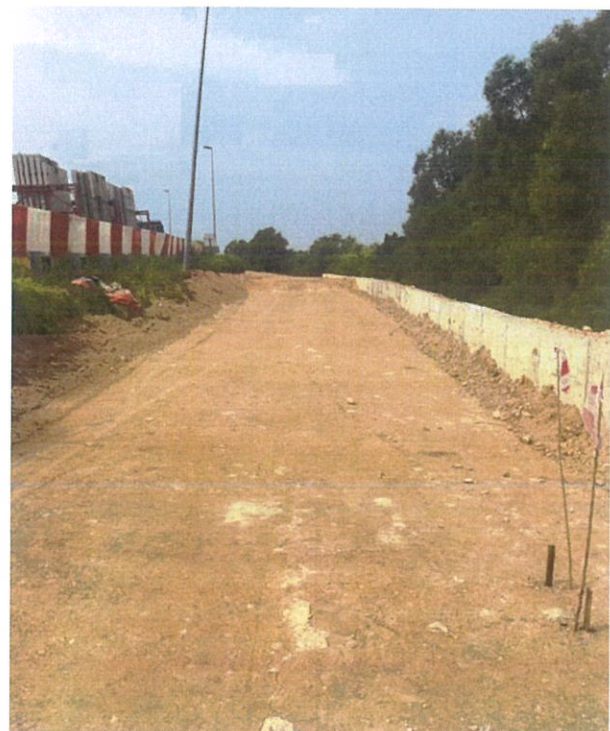
PHOTO 12: Earthworks in progress at CH C (SKVE)
