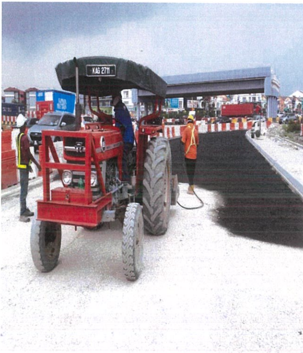
PHOTO 5: Preparation for pavement works in progress at CH B
