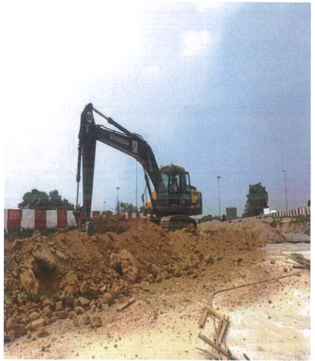
PHOTO 2: Pile Embankment - Excavation & backfilling works in progress at zone 3 SKVE
