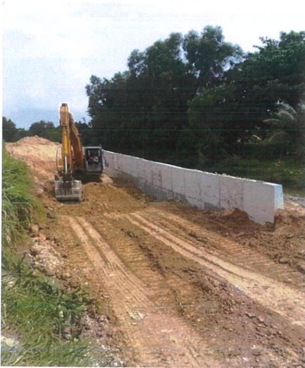
PHOTO 9 : RC Wall completed at CH C (SKVE) - Earthwork in progress
