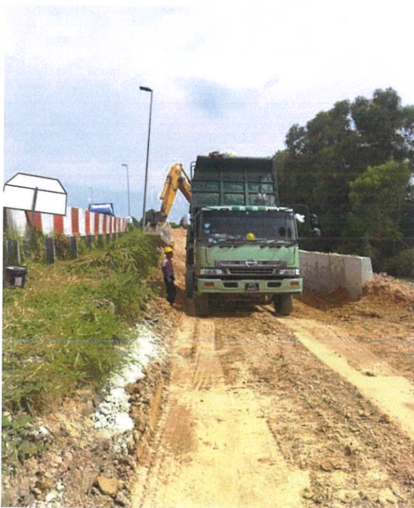
PHOTO 11: Earthworks in progress at CH C (SKVE)
