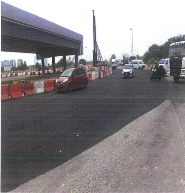
PHOTO 13: Resurface roundabout area in progress
