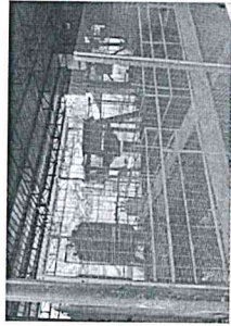
3 STAGE INITIAL SEPARATION TANK 70M 2 BATCHING CAPACITY
